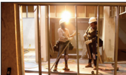
3 out of the 7 women are currently employed as apprentice carpenters.
